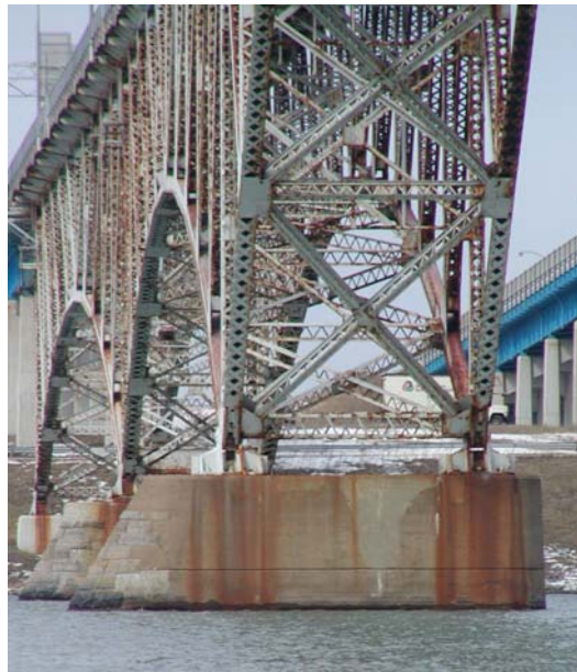
Figure 1. Typical Steel Truss Pier
